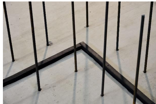
Fastening with swelling tape adhesive
