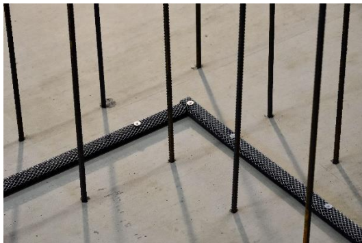
Fastening with swelling tape grid
